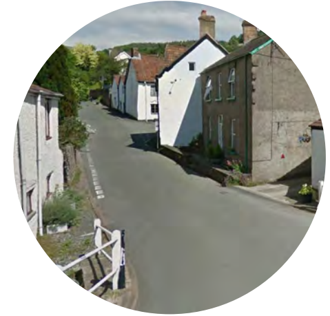
Limited footway provision, Brockwier
