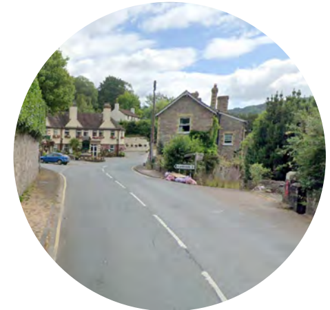
PROW without on crossing A466, north of Tintern
